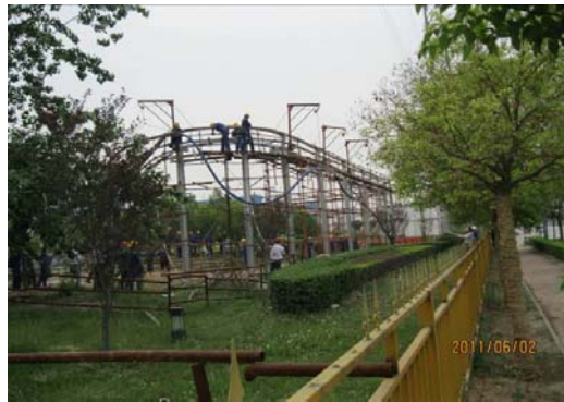
Fig.11. The 360m/10kA DC HTS cable under installation.
