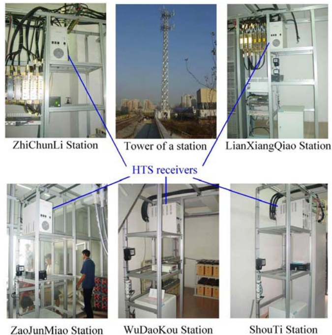
Fig.21. Superconducting filter system operating in various base stations of the demonstration base for mobile telecommunications application in Beijing.
