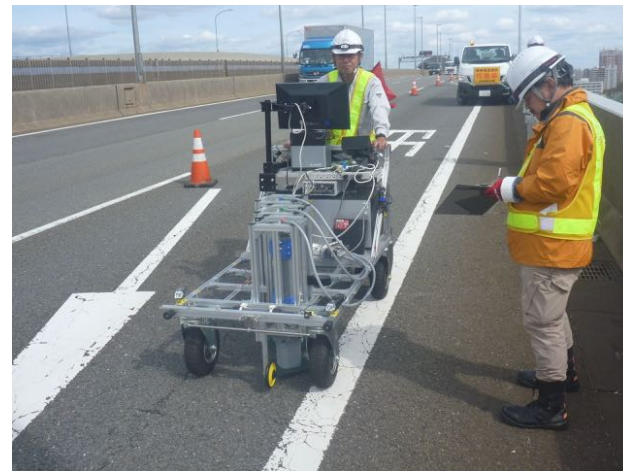
Field test on expressway bridge (Oct. 2018)
