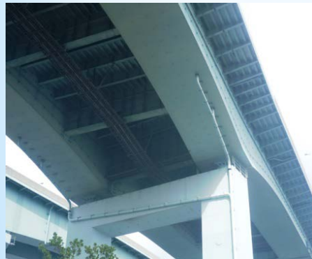
Orthotropic steel deck bridge (Hanshin expressway)
