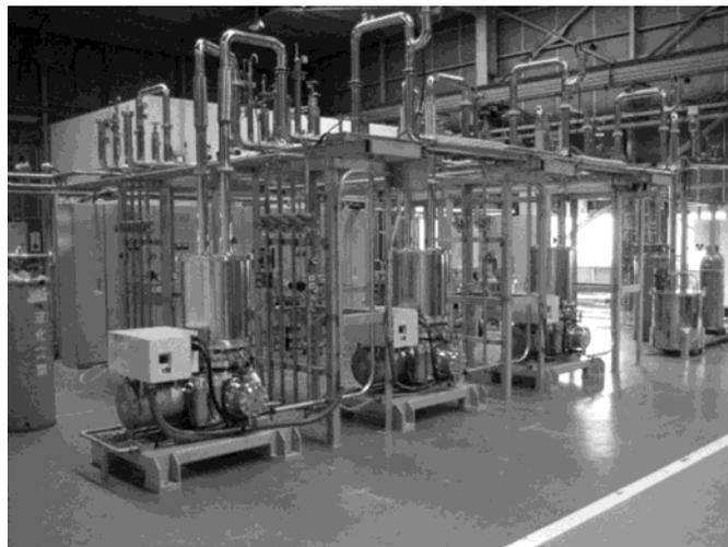
Fig. 12. Overview of the cooling system constructed at Mayekawa's factory. This cooling system has the same configuration as that for Asahi substation, though the number of refrigerator is three instead of six.
