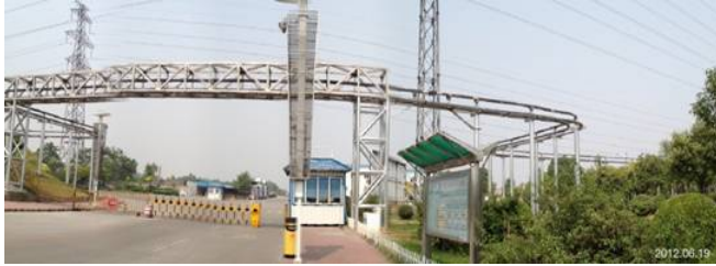
Fig.4. An overview of the 10kA HTS DC power cable after installation.
