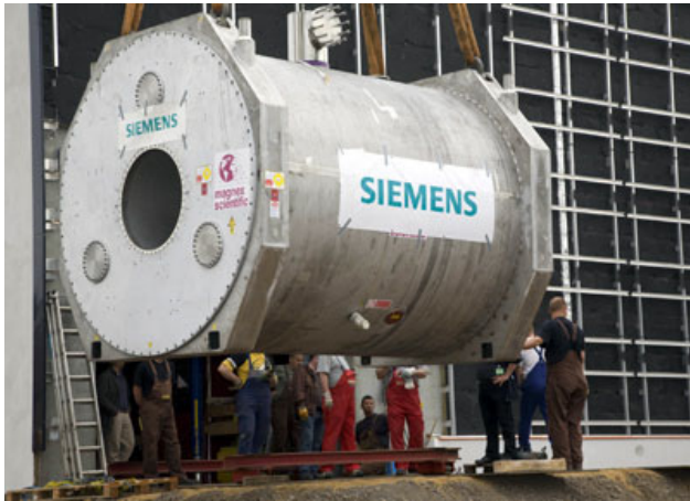
9.4 T 90 cm 54 tons MRI PET Scanner in operation at Julich, Germany
