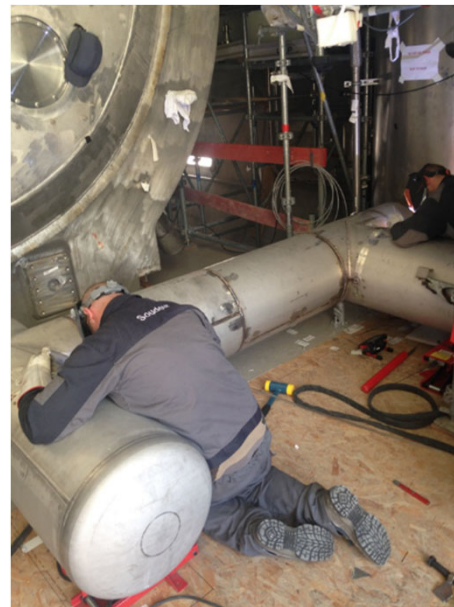
Vacuum vessel welding
