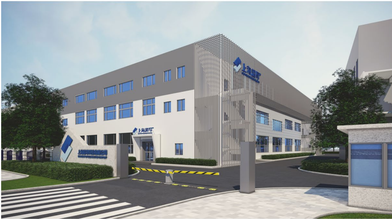
Renovation Design and Work Underway
